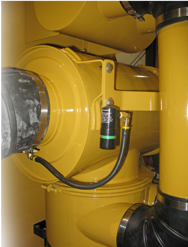
Figure 5-5-15 Air Cleaner Indicator
