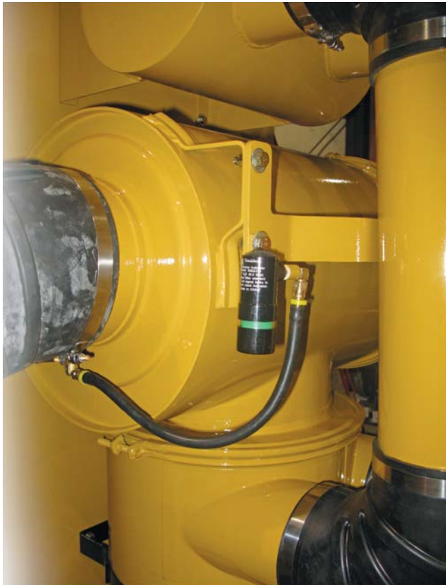
Figure 5-5-15 Air Cleaner Indicator
