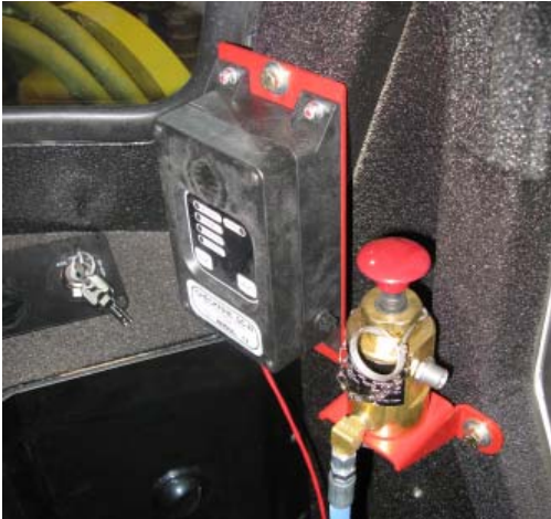
Figure 3-35 Fire Suppression System Shown with Automatic Detection and Activation System
