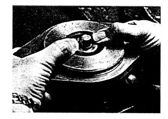
Using Seal Driver DAP24-64 drive the seal into the adapter.
