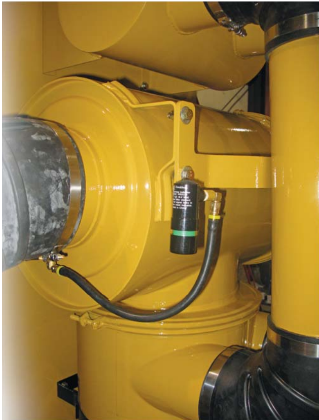
Figure 15 Air Cleaner Indicator
