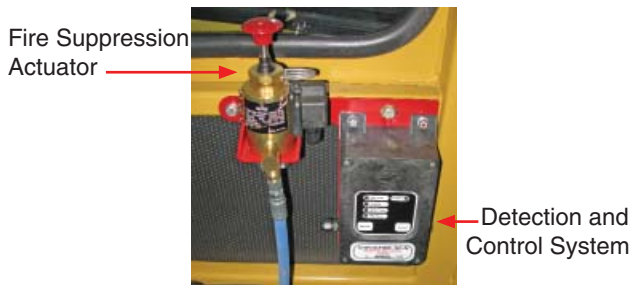
Figure 11 - Fire Suppression System
