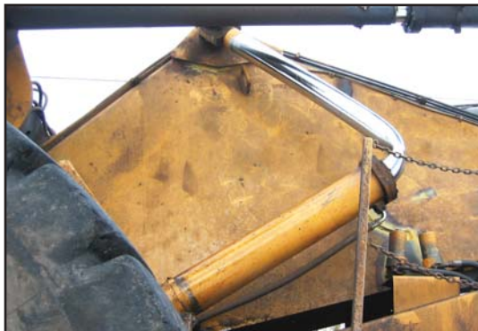
Figure 3. Damaged cylinder on log stacker
